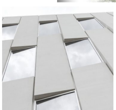
Above: 1200 Intrepid Avenue, Philadelphia, PA Navy Yard Left: Detail of faceted panel with window integration
