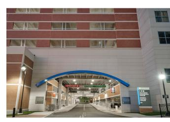
"FROM THE BEGINNING, CHRISTIANACARE WAS DEDICATED TO USING A PRECAST CONCRETE STRUCTURAL SYSTEM WITH THIN BRICK TO MATCH THE RECENTLY COMPLETED ADJACENT HOSPITAL TOWER EXPANSION PROJECT."
