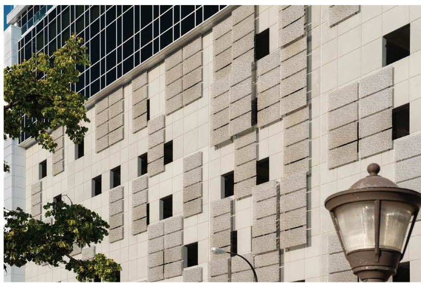
Above: 500 Pearl Street, Buffalo, NY finished building.
