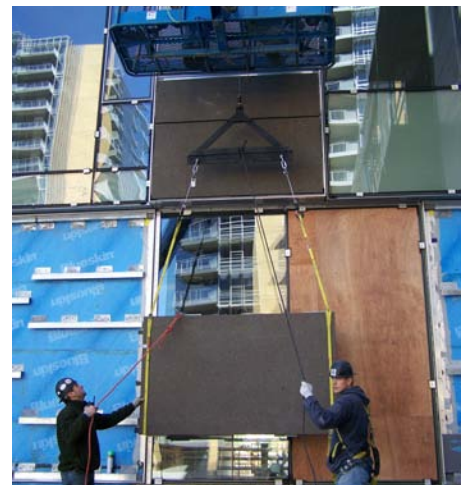
Manual installation of light-weight panel over insulation
