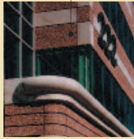
Water wash, acid etch, medium blast.
