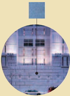
Formliner acid etch, water washed.
