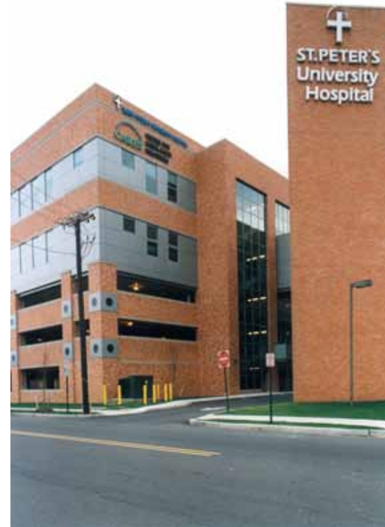
Decorative medallions at the corners of the new structure’s parking lot match the exposed concrete of the surgery center above, while brick blends with the existing medical center at right. Photo: JP McKenna, Architectural Photography
