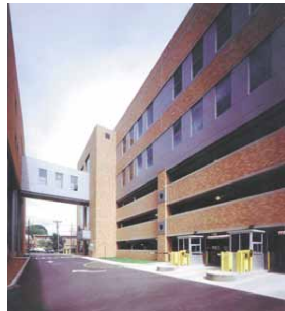
The need to provide a pedestrian link from the new addition to the existing facility played a major role in the decision to place the surgery center atop the new parking structure. Photo: JP McKenna, Architectural Photography
