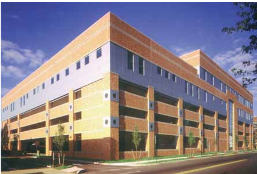
St. Peter’s Medical Center in New Brunswick, N.J., constructed its new Ambulatory Surgery Center atop its new parking structure using a precast concrete structural system for both. American Medical Building’s development approach created efficiencies in time, cost and access for the hospital. Photo: JP McKenna, Architectural Photography
