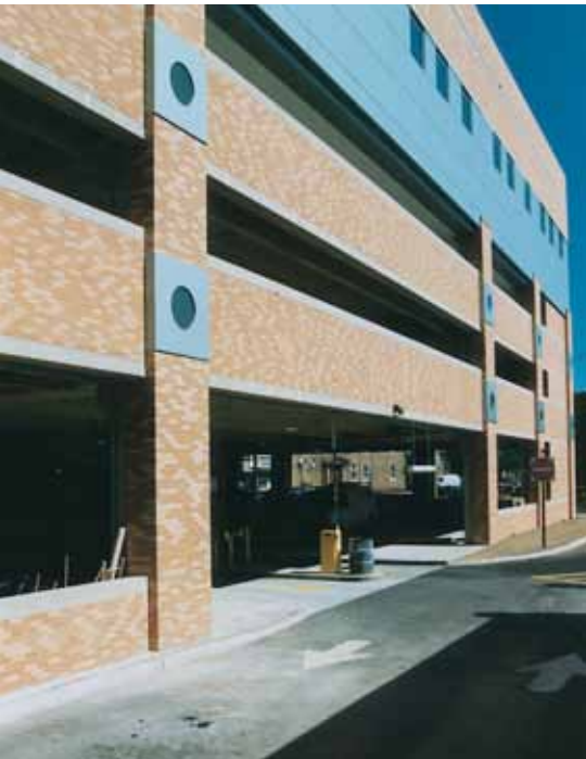
The parking structure was constructed with long-span concrete framing members, which alleviated an acute parking shortage for the land-locked medical center. Photo: Robert Meier, Architectural Photography
