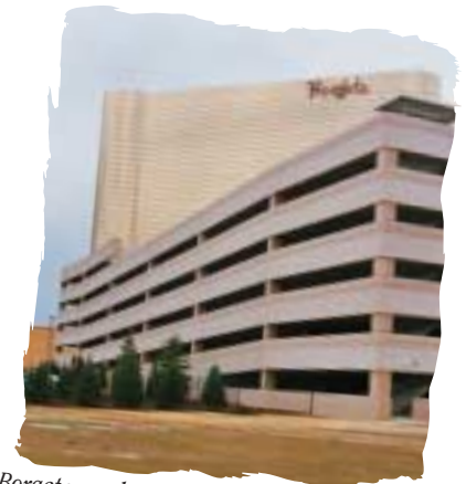
Borgata employee parking garage provides safe parking for Borgata's 4,000-person staff.
