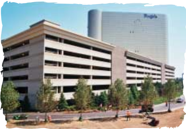
The Borgata Casino parking garage was also a High Concrete project.
