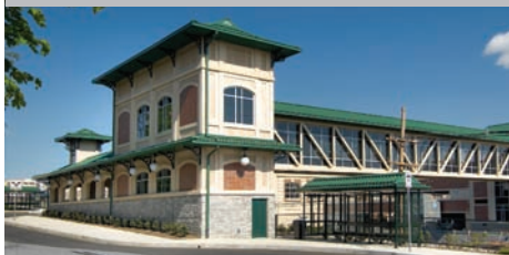
Formliner created the distinctive "retro" look of the wall panels on the commuter station.
