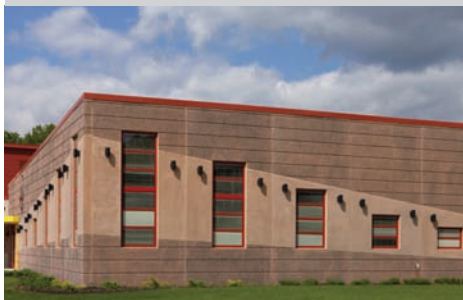
Exposed aggregates and tile accents create a dynamic exterior.
