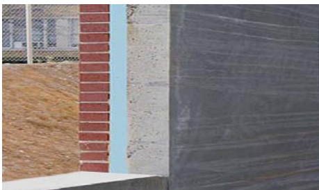
Sandwich precast wall panels provide edge-to-edge insulation for "ci" as defined by ASHRAE 90.1.
