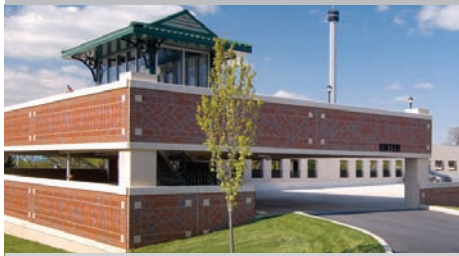
Thin brick captured the spirit of the period brickwork of the nearby historic press building that was restored in the project.
